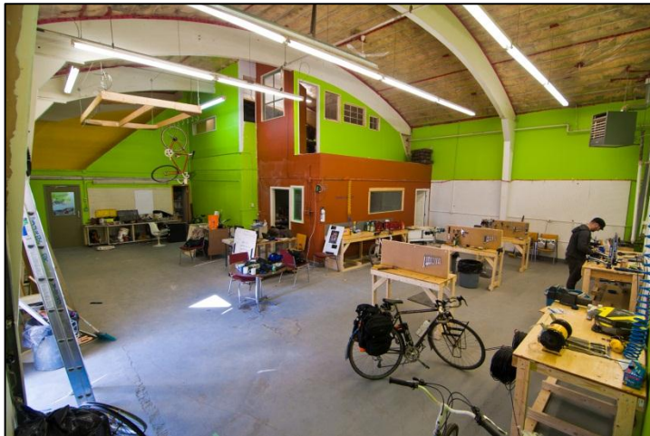
BikeWorks North undergoing renovations
